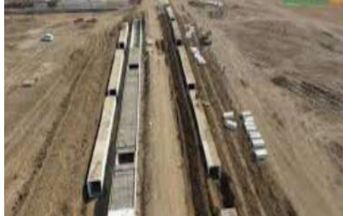
Drainage network construction
