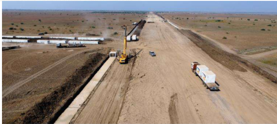
Power Duct Laying In Progress. - H-1
