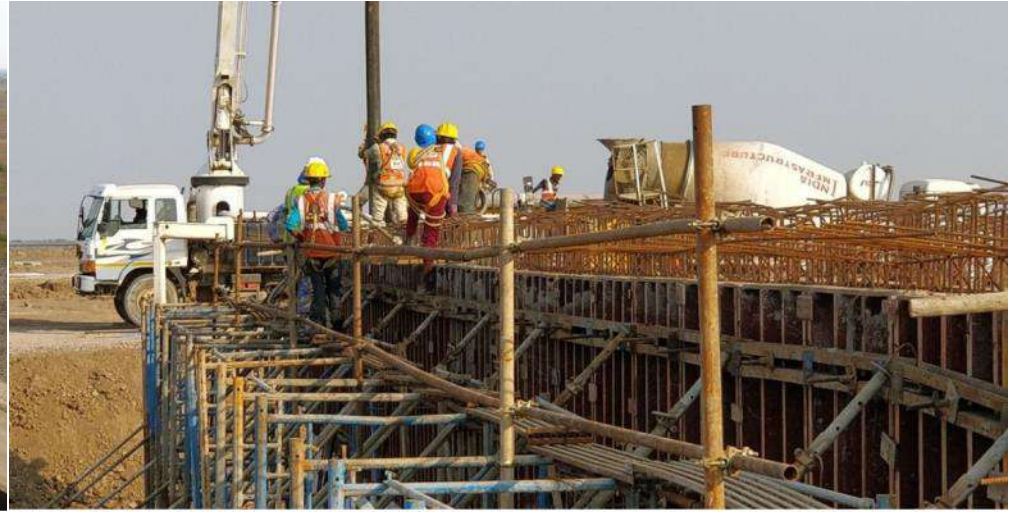
E-3 BRIDGE: SUBSTRUCTURE CONCRETING
