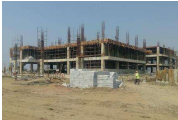
BEC 2 nd Slab Shuttering
