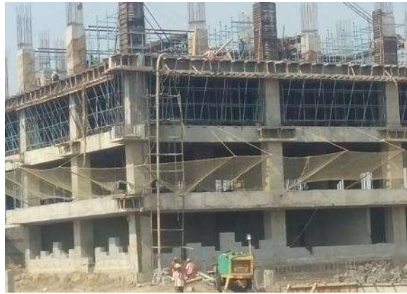
SPV Building 4 th floor column progress
