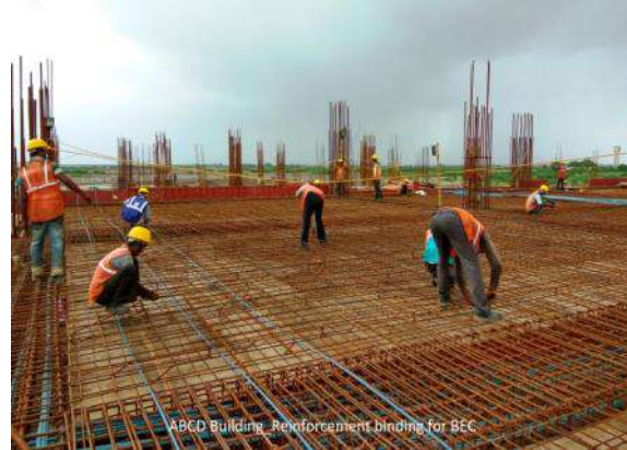
Reinforcement for BEC Slab
